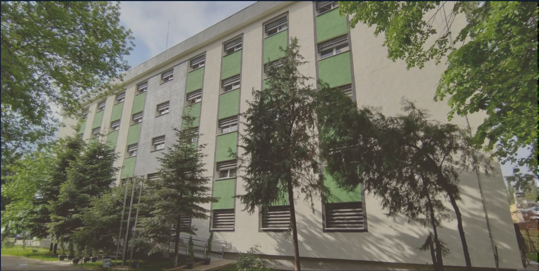
Ilfov County Gendarmerie Inspectorate
